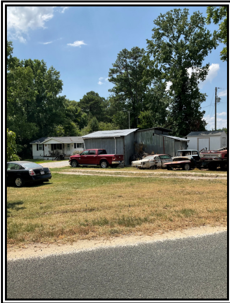
Single-Family residence to the adjacent south on Parrish Road
