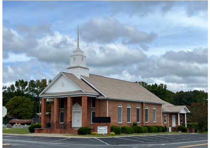
Historic communities generally have a history of residential, commercial and institutional uses. Christian Light Christian Church pictured above is an example of the type and scale of development in these areas.
