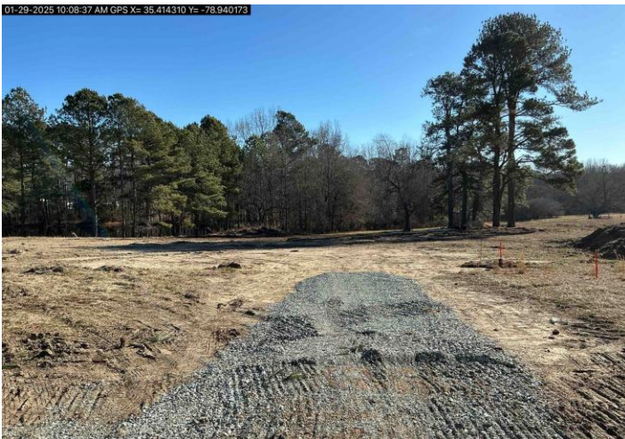
Site/131 Griffin Rd.
