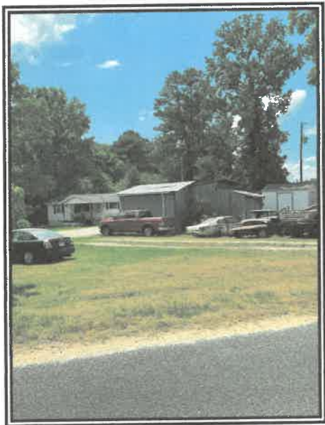
Single-Family residence to the adjacent south on Parrish Road
