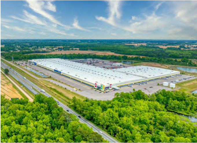
Furniture retailer Rooms to Go recently announced plans to expand its 1,450,000 square foot distribution center along I-95.
