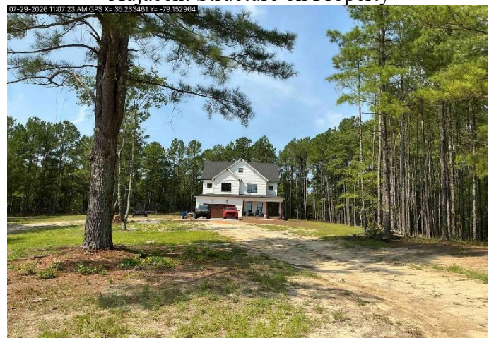
Adjacent Structure on Property
