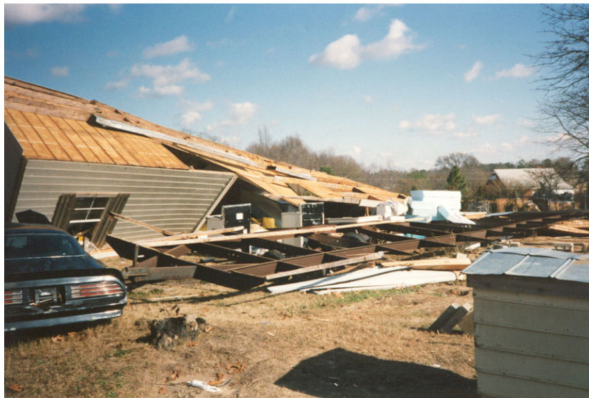
A mobile home in Harnett County following a tornado in January of 1995
